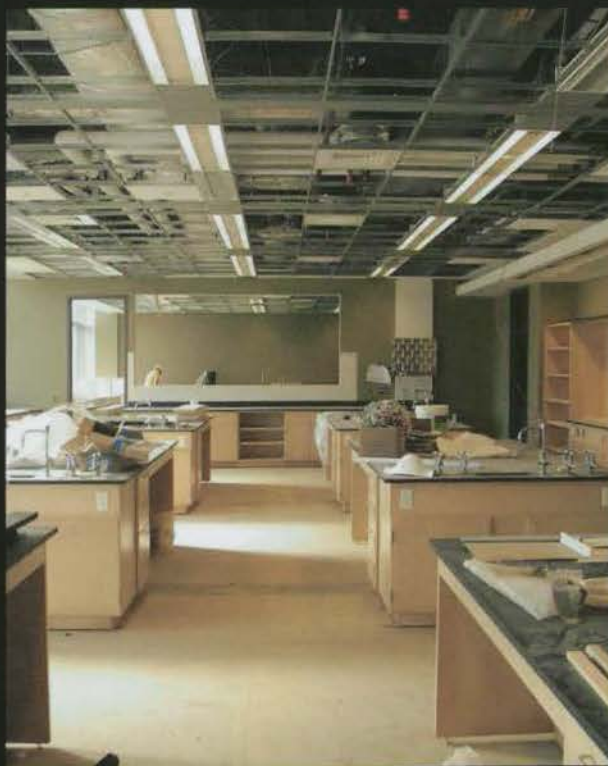
Above: Earlier this year, the laboratory is still under construction.
