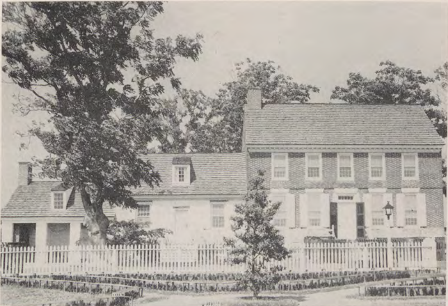
The John Dickinson Mansion, shown here as it stands today restored after years of decay and neglect, is a fine example of Delaware
