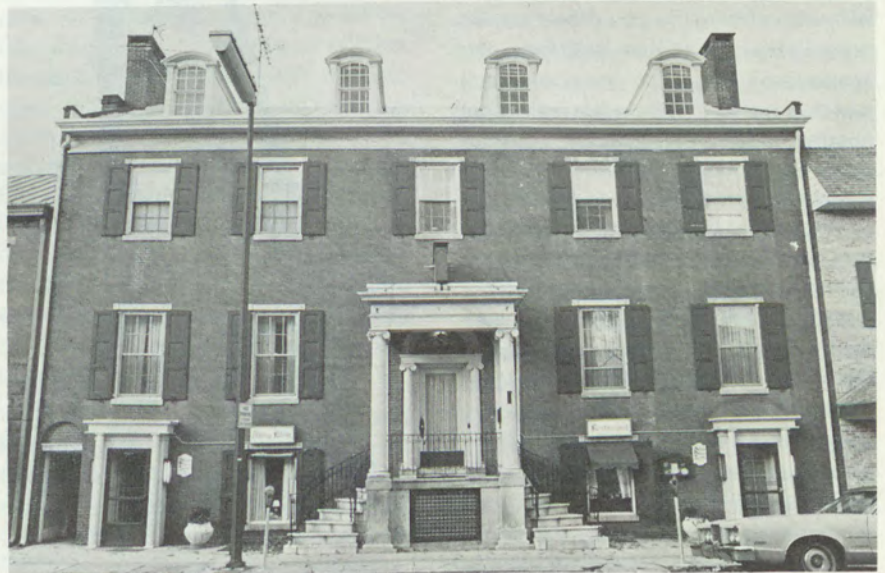
143 High St. — Typical 19th century adaptation of Georgian style, as well as Greek Revival elements.
