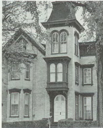
315 N. Hanover St. — Mid-Victorian cottage built in two sections, 1890 and 1920.
