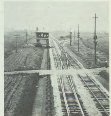
A view of the interlocking plant at "QN" tower, the author's place of employment.
