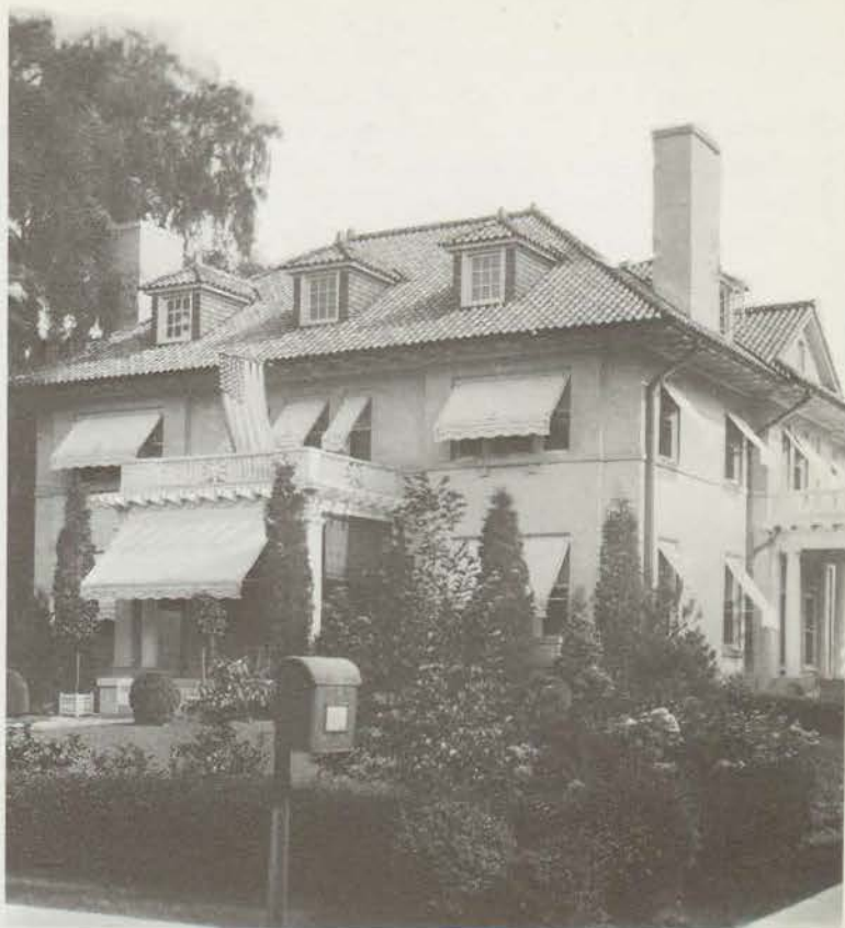
The same corner only a few years later, as it appears today: the Admissions House, formerly Alpha Chi Rho. Photo by A. A. Line.
