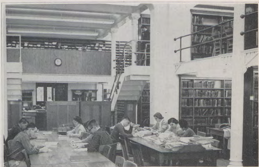
Main Reading Room of the Library as it looks today after extension of the balcony into a U-shaped deck and the installation of two stairways. New fluorescent fixtures have increased the lighting.
