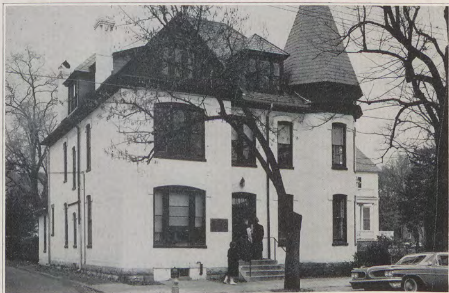
After extensive alterations and given a new name, the old Methodist church house (above) has become the new home of the Department of Education and Psychology.
