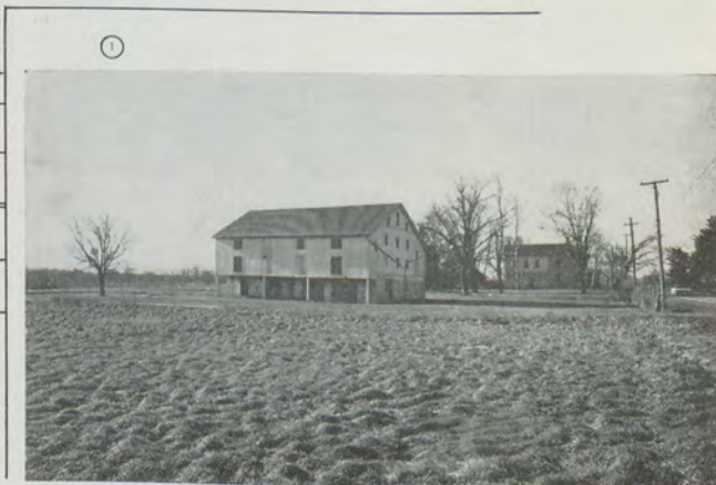
A view of the 65-acre tract showing the farmhouse and barn.
