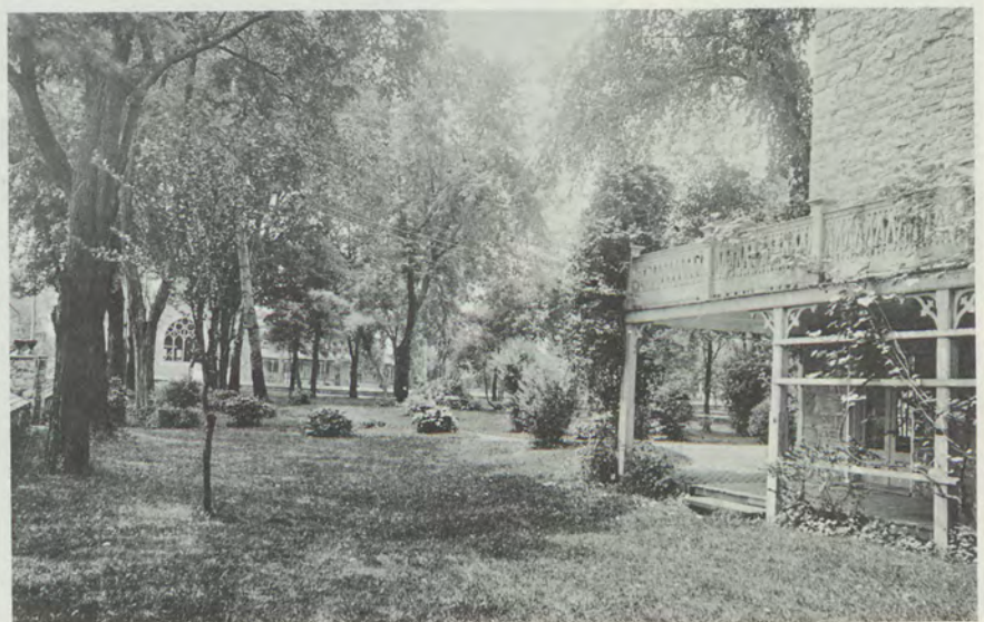
From the West street side of Old East, now the Bernard Center, it was possible to look toward Allison Church, then on the southwest corner of West and High streets (right). What is now the president's house is visible beyond it. This end of Old East was the president's home until 1890. This Allison Church burned in 1954.
