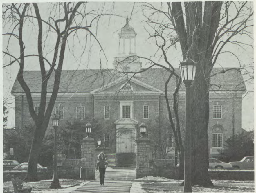
Alumni gymnasium prior to the beginning of the renovation.
