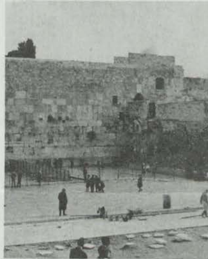
The Kotel or western wall.
